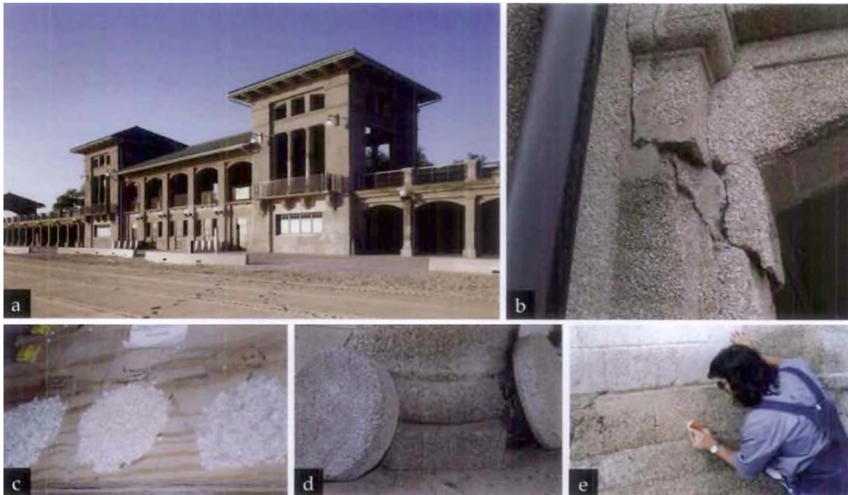
Figure 17. (a) The 63rd Street Beach House was constructed on the shoreline of Chicago in 1919. The highly exposed aggregate concrete of the exterior walls of the beach house was used for many buildings in the Chicago parks as an alternative to more expensive stone construction. Photo: Leslie Schwartz Photography. (b) Concrete deterioration included cracking, spalling, and delamination caused by corrosion of embedded reinforcing steel and concrete damage due to cyclic freezing and thawing. (c) Various sizes and types of aggregates were reviewed for matching to the original concrete materials. (d) Mock-ups of the concrete repair mix were prepared for comparison to the original concrete. Considerations included aggregate type and size, cement color, proportions, aggregate exposure, and surface finish. (e) The craftsman finished the surface to replicate the original appearance in a mock-up on the structure. Here, he used a nylon bristle brush to remove loose paste and expose the aggregate, creating a variable surface to match the adjacent original concrete.
