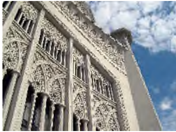
Figure 4. The highly ornamental concrete panels on the exterior facade of the Baha'i House of Worship in Wilmette, Illinois, illustrate the work of fabricator John J. Earley, known as "the man who made concrete beautiful."
