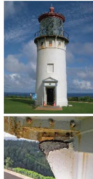
Figure 12. The concrete lighthouse at the Kilauea Point Light Station, Kilauea, Kauai, Hawaii, was constructed circa 1913. The concrete, which was a good quality, high strength mix for its day, is in good condition after almost one hundred years in service. Deterioration in the form of spalling related to corrosion of embedded reinforcing steel has occurred primarily in areas of higher ornamentation such as projecting bands and brackets (see close-up photo).
