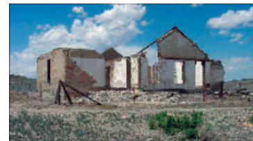
Figure 2. Chatterton House was the home of the post trader at Fort Fred Steel in Wyoming, one of several forts established in the 1860s to protect the Union Pacific Railroad. The walls of the post trader's house were built using stone aggregate and lime, without cement. The use of this material presents special preservation challenges.
