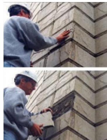
Figures 14. Layers of architectural concrete that have debonded (spalled) from the surface were removed from a historic water tank during
