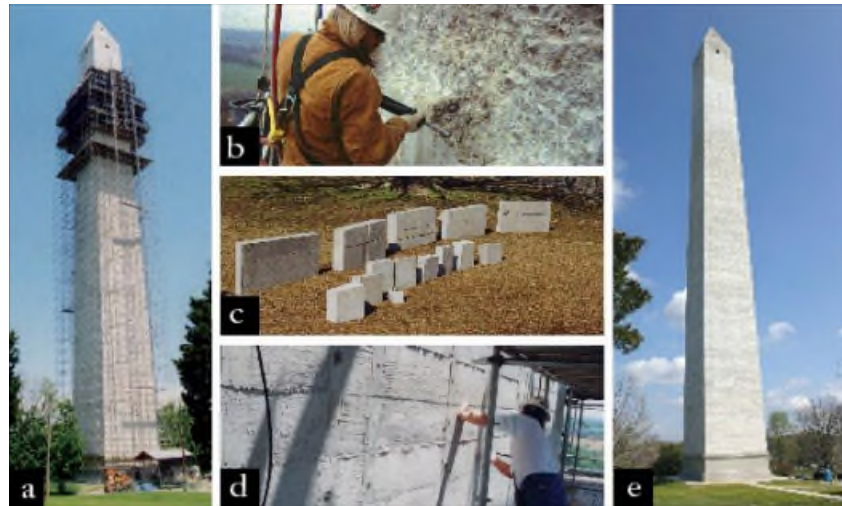
Figure 20. (a) The Jefferson Davis Memorial in Fairview, Kentucky, constructed from 1917-1924, is 351 feet tall and constructed of unreinforced concrete. The walls of the memorial are 8 feet thick at the base and 2 feet thick at the top of the wall. Access to the monument for investigation was provided by rappelling techniques, while ground supported and suspended scaffolding was used to access the exterior during repairs. (b) The concrete was severely deteriorated at isolated locations, with spalling and damage from cyclic freezing and thawing of entrapped water. In addition, previous repairs were at the end of their service life and removal of deteriorated concrete and failed previous repairs was required. Light duty chipping hammers were used to avoid damage to adjacent material when removing deteriorated concrete to the level of sound concrete. (c) Field samples were performed to match the color, finish, and texture of the original concrete. A challenge in matching of historic concrete is achieving variability of appearance. (d) The completed surface after repairs exhibits intentional variability of the concrete surface to match the appearance of the original concrete. Some formwork imperfections that would normally be removed by finishing were intentionally left in place, to replicate the highly variable finish of the original concrete. (e) The Jefferson Davis Memorial after completion of repairs in 2004. Photo e: Joseph Lenzi, Senler, Campbell & Associates, Inc.
