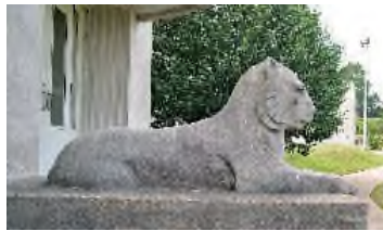
Figure 7. Detailed bas-reliefs as well as sculptures, such as this lion at the Bailey Magnet School, could be used as ornamentation on concrete buildings. Sculptural concrete elements were typically cast in molds.
