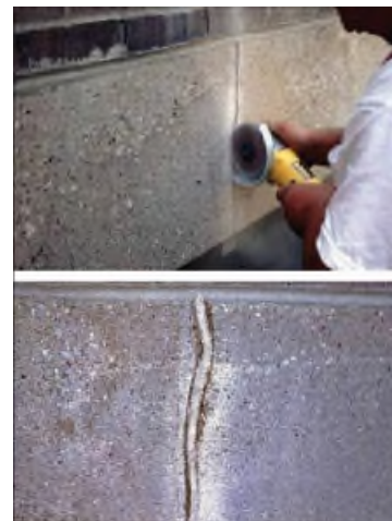
Figure 19. A high-speed grinder is used to widen a crack in preparation for installation of a sealant. This process is called "routing." After the crack is prepared, the sealant is installed to prevent moisture infiltration through the crack. Although sealant repairs can provide a durable, watertight repair for moving cracks, they tend to be very visible.
