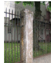
Figure 15. Evidence of moisture movement through concrete is apparent in the form of mineral deposits on the concrete surface. Cyclic freezing and thawing of entrapped moisture, and corrosion of embedded reinforcement, have also contributed to deterioration of the concrete column on this fence at Crocker Field in Fitchburg, Massachusetts, designed by the Olmsted Brothers.
