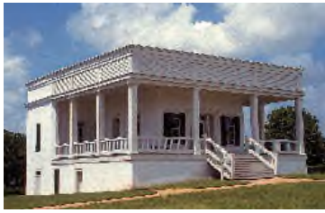
Figure 1. The Sebastopol House in Seguin, Texas, is an 1856 Greek Revival-style house constructed of lime concrete. Lime concrete or "limecrete" was a popular construction material, as it could be made inexpensively from local materials. By 1900, the town had approximately ninety limecrete structures, twenty of which remain. Photo: Texas Parks and Wildlife Department.
